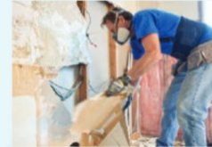
Drywall & Cement Sheets
