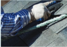
Roof Shingles & Siding
